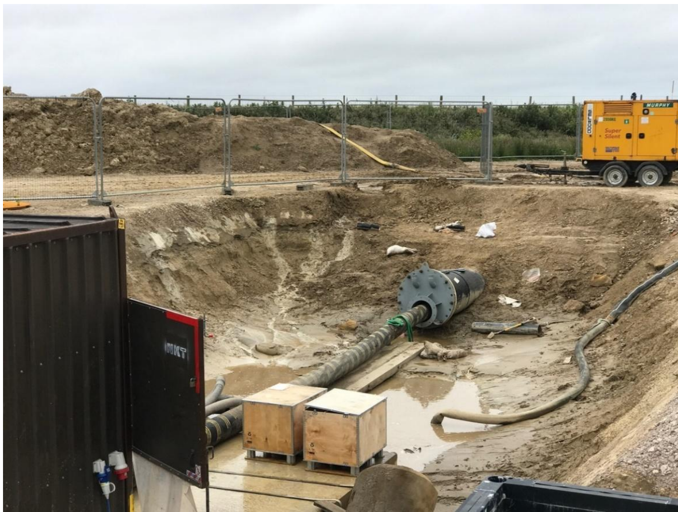
Plate 4.4 Example of an HDD sealing plate at onshore end (Walney Extension Offshore Wind Farm)
